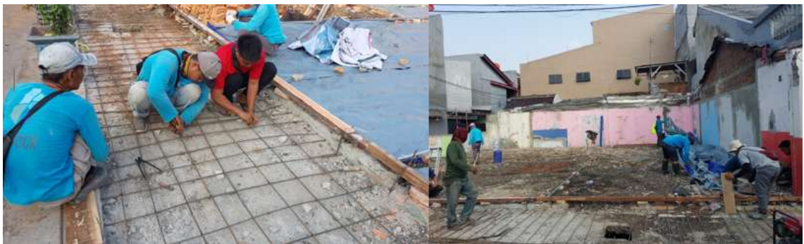
Figure 6. The process of assembling reinforcement in the culvert area
