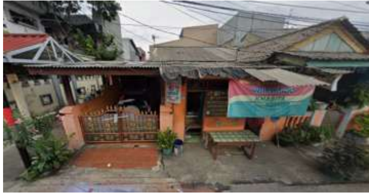
Figure 1. Existing Building Condition Prior to Redevelopment as a Church Parking Area
