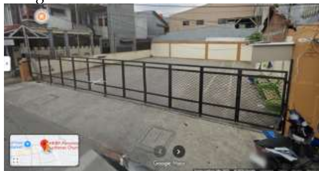
Figure 9. Finishing the parking area of the HKBP Perumnas Klender church Sumber: ( https://maps.app.goo.gl/wM4iWY8f3MpK4jxn7 )
