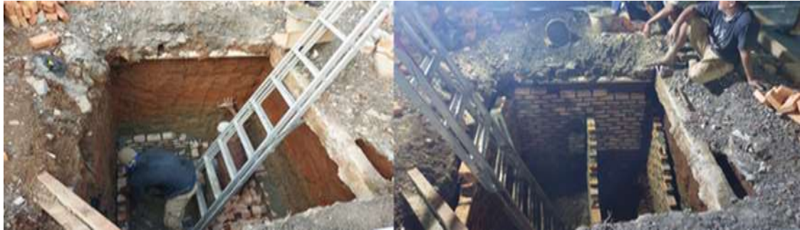
Figure 7. Installation of septic tanks in the parking area of HKBP Perumnas Klender
