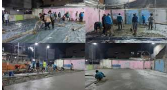
Figure 8. The process of casting the parking area of HKBP Perumnas Klender.
