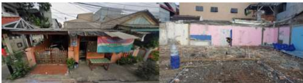
Figure 4. Dismantling of existing buildings and soil compaction process using stampers
