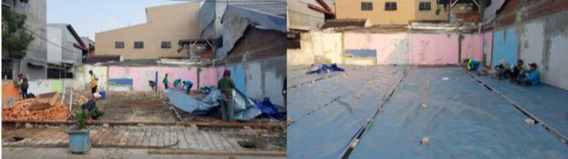
Figure 5. The process of installing the tarpaulin in the casting zone and levelling determination before casting
